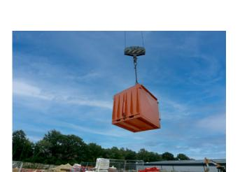
Designed for the safe transportation of palletized bricks and blocks on both standard and telescopic crane forks. The 1058.7 can be used with crane forks from any manufacturerer meaning you can buy just the cage and use your existing forks. The system has major safety benefits over the traditional use of safety nets.
